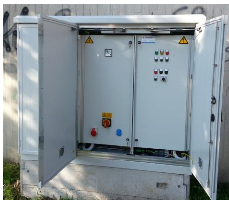
Interior door, door lock, contact switch and electric socket
